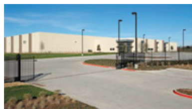
Stream Realty Data Center
